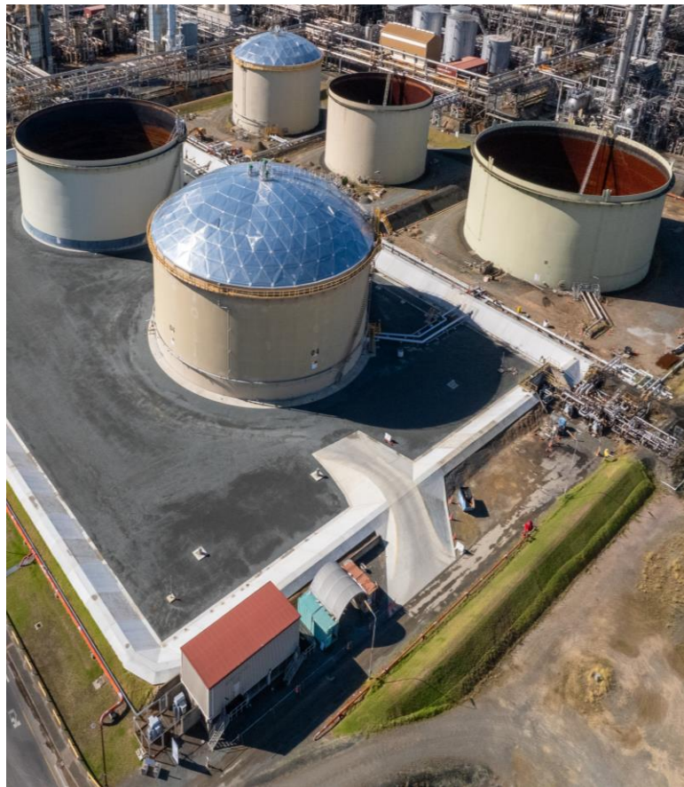
Crude oil to jet fuel tank conversion – new geodesic roof
