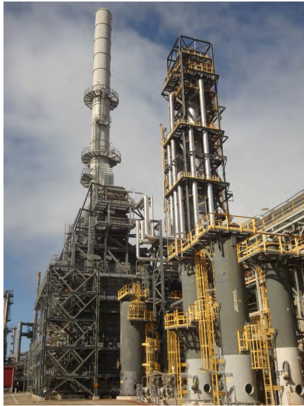
Figure 11: E-Block Commissioned in 2015 remains complete and under a Nitrogen purge.
