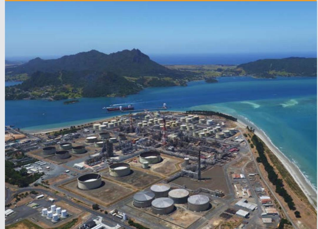
Refining NZ is proposing changes to Whangarei's harbour entrance which would allow larger crude cargoes to be brought into Marsden Point. Larger ships come to the Refinery under loaded because the shipping channel is not deep enough. Loading them to full capacity (around one million barrels) would require deepening and realigning the shipping channel through dredging.
